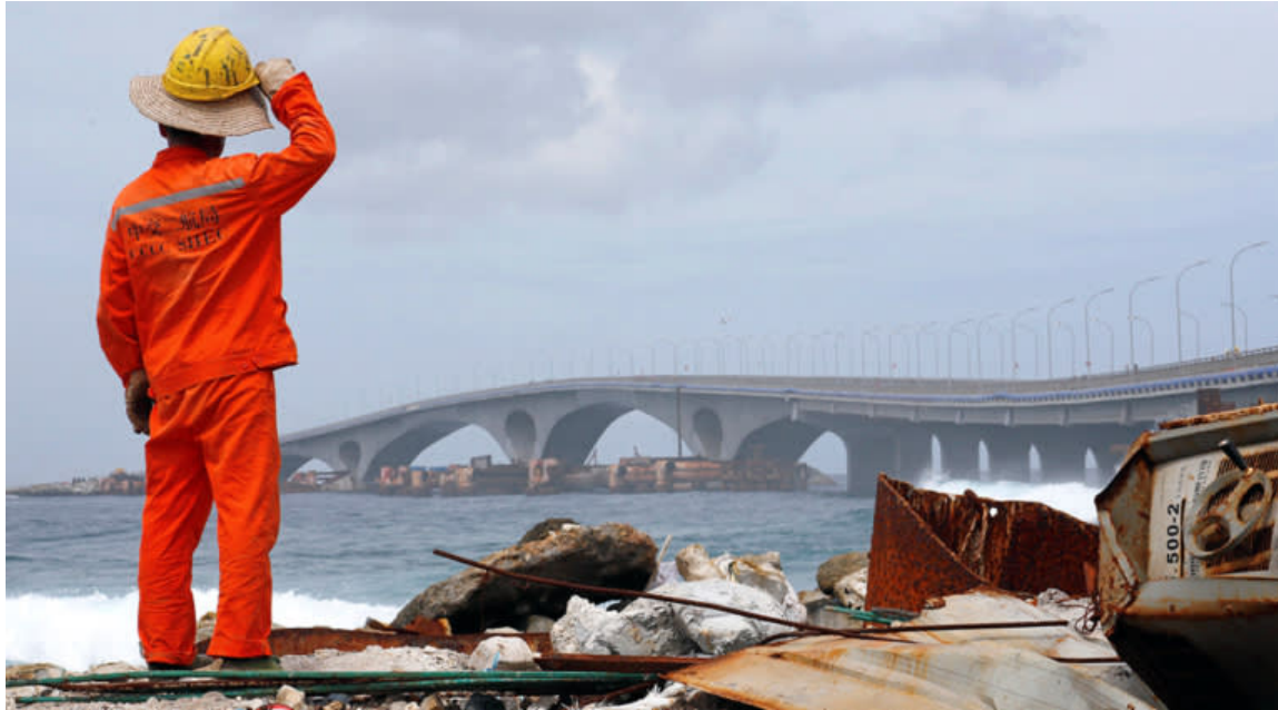
A construction worker gazes at the China-funded Sinamale bridge in Male, Maldives, in September 2018. © Reuters
